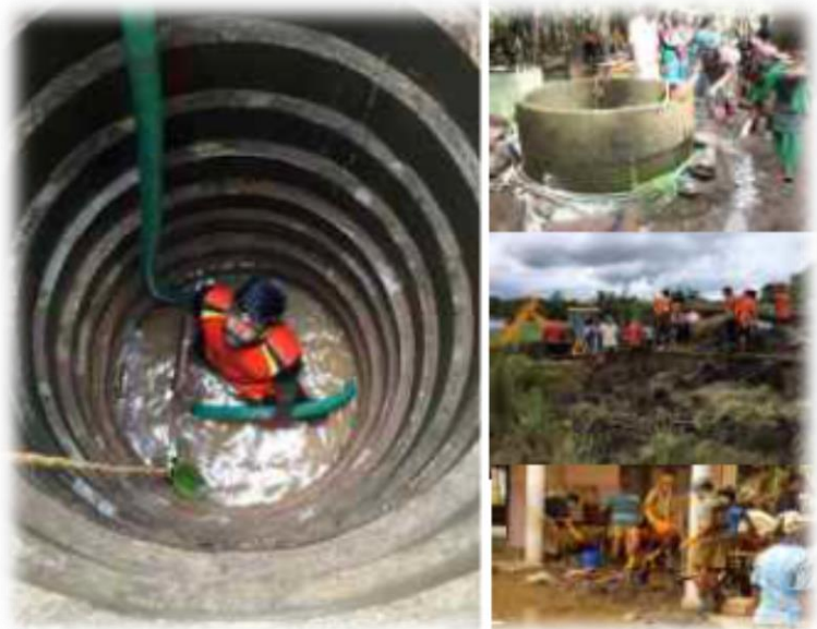
Pic 15. Volunteers pumped out slush and contaminated water from wells, chlorinated them, and cleaned other public places.
